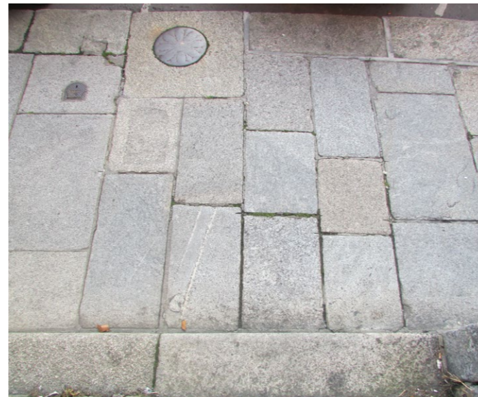
Historic pavements with cellar covers intact
