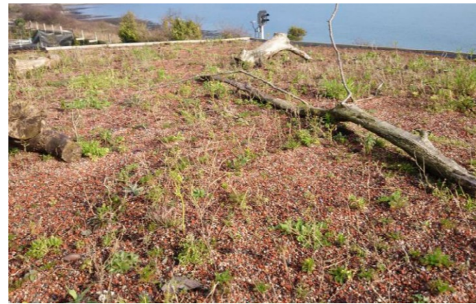
Functional inaccessible Brown roof systems
