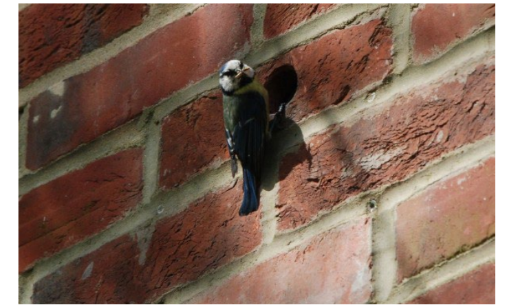
Subtle brick specials with cavity for birds or bats
