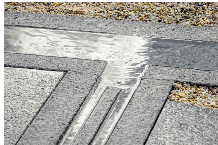
--- Dished granite surface gully
