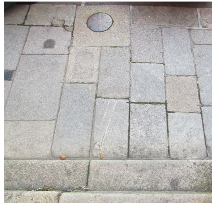
Existing historic pavement to be retained
